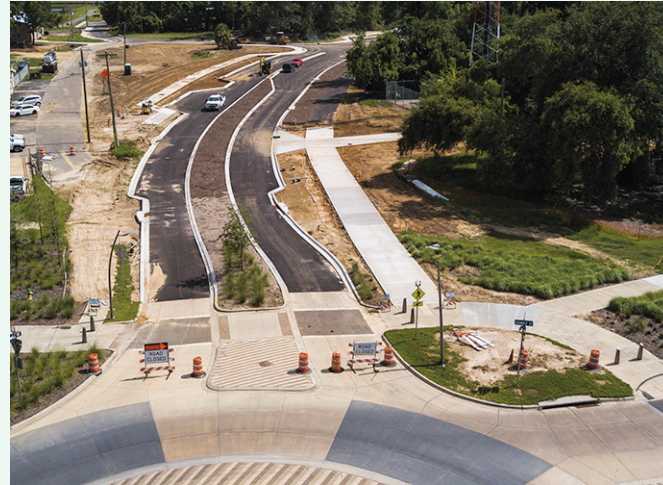
FAMU Way Extension Project (Phase 3)
