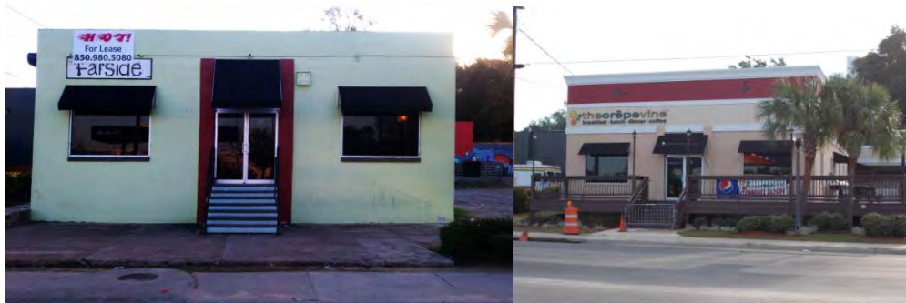
The Crepevine Restaurant before renovations (left) and after renovations (right).
