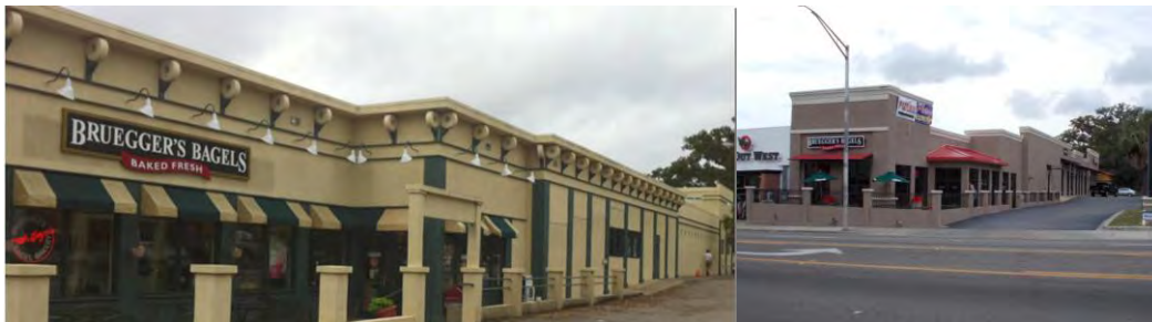
The Merchant’s Row at Midtown before renovations (left) and after renovations (right).
